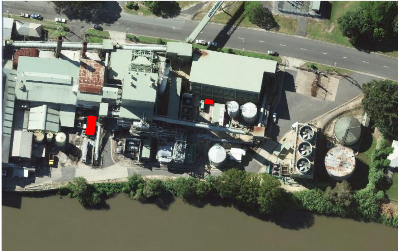
Figure 1. Site Layout of Condong Cogeneration Plant indicating primary Chemical Storage Areas in red.
