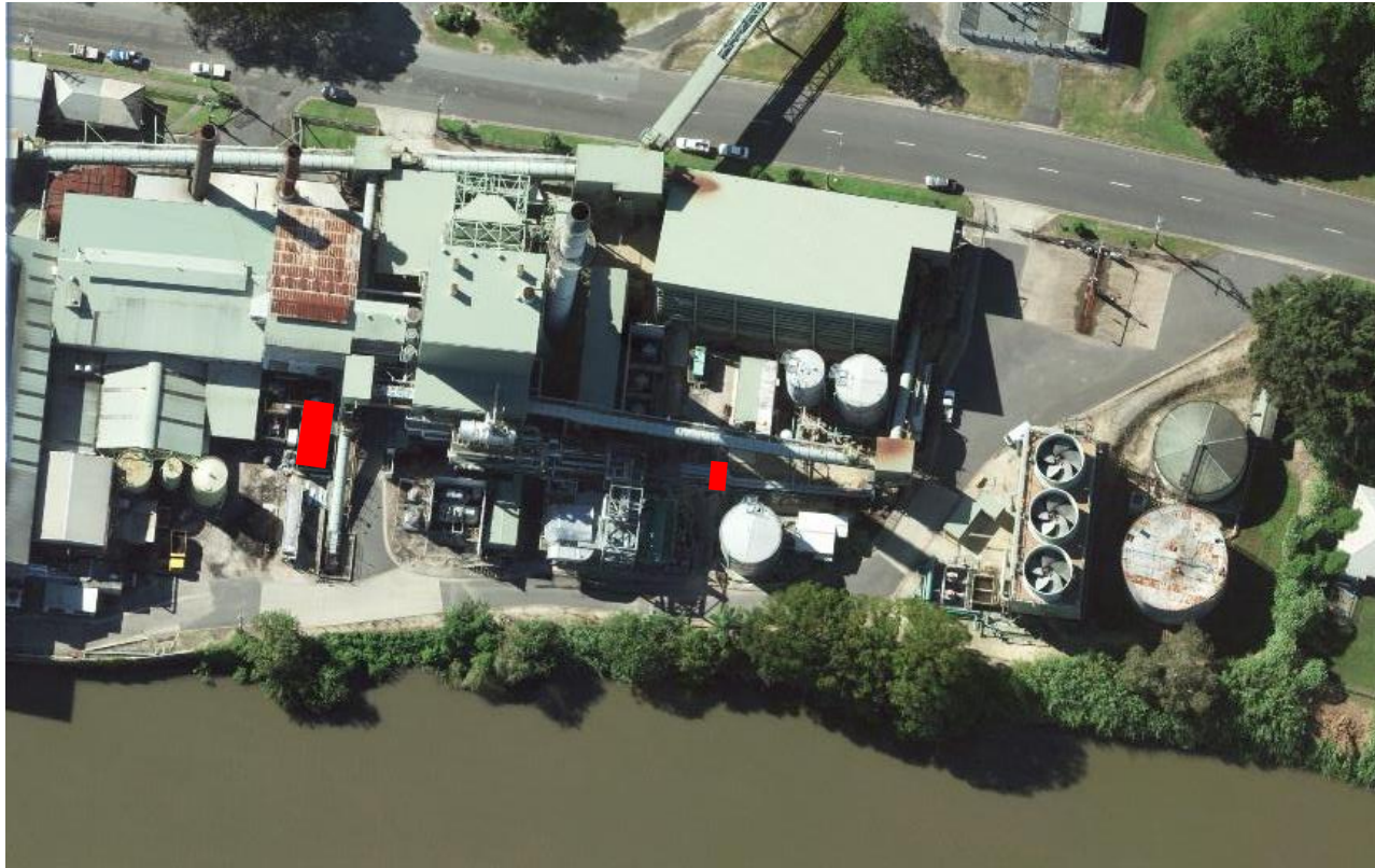
Figure 1. Site Layout of Condong Cogeneration Plant indicating primary Chemical Storage Areas in red.
